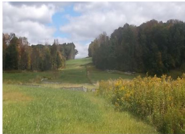
TGP Right-of-Way Post-Construction 9/26/2013
